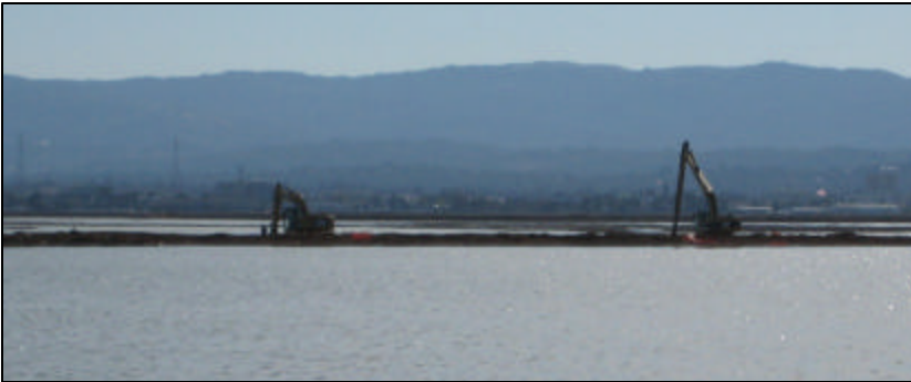
Progress continues on the levee breaches on Middle Bair Island
